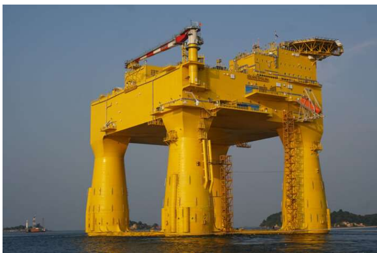
Figur 4.2-Gravitationsbaserad struktur under transport
